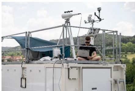
On the roof of the QuBUS, which is located on the premises of the Fraunhofer IOF, is the unit for receiving the quantum keys sent via free-space from the Jena public utility. © Fraunhofer IOF
